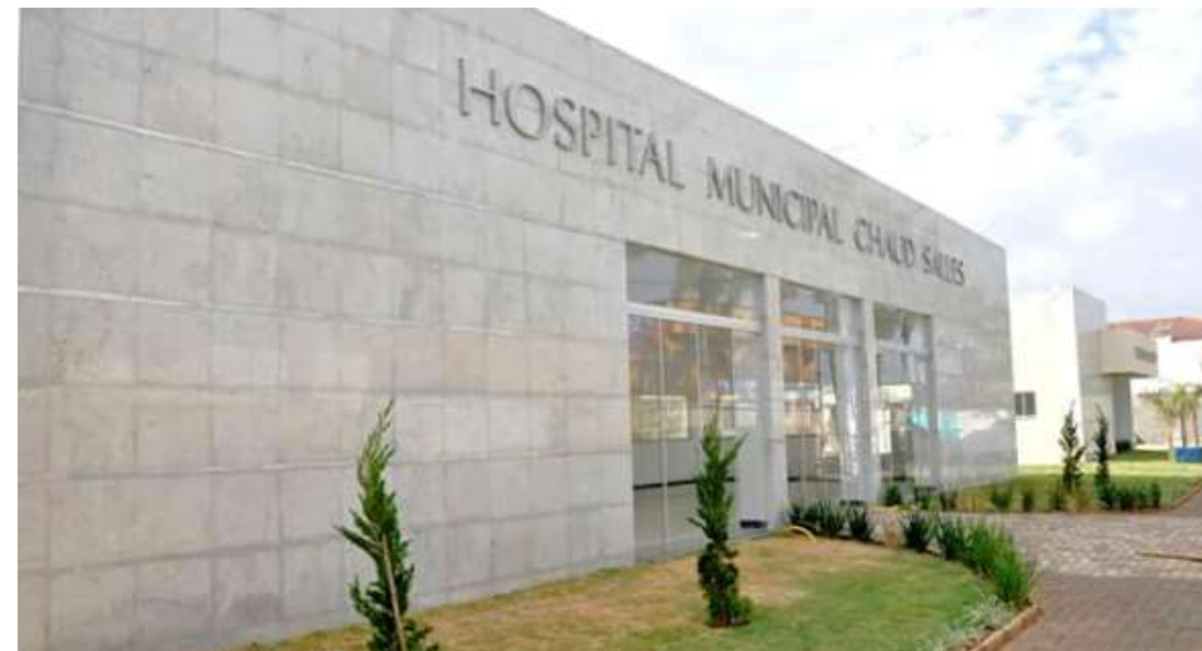
Hospital Municipal Chaud Salles – Cristalina - GO
